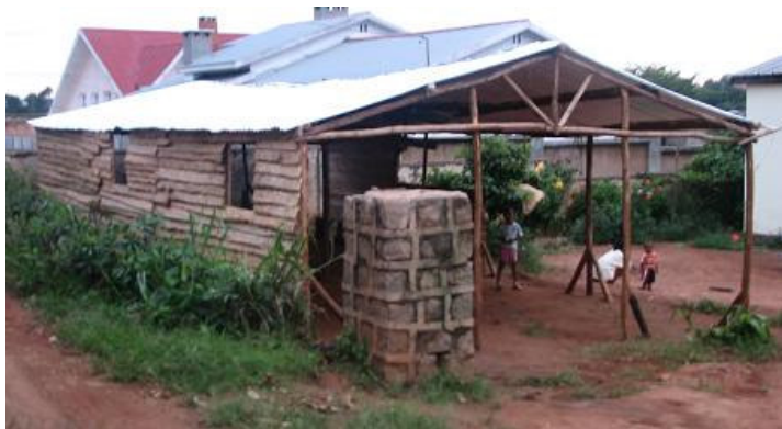
← Photo at Left: Here is the new church still under construction
